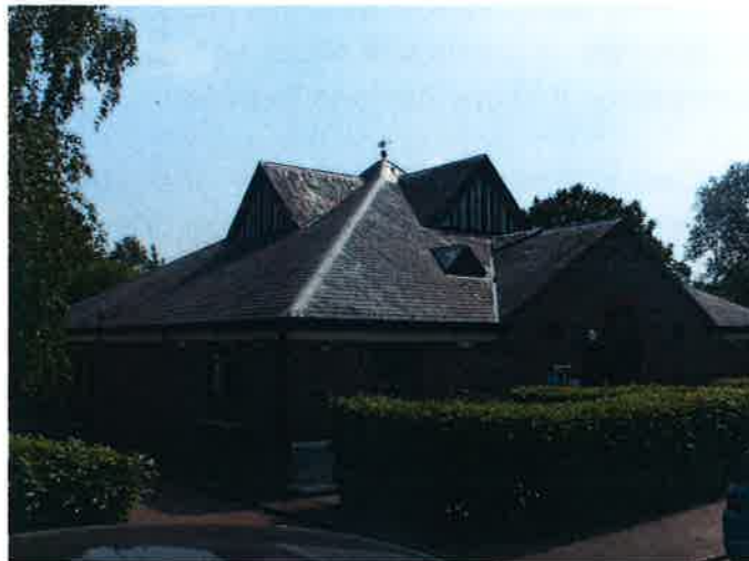
North Heath Hall, North Heath Lane.
